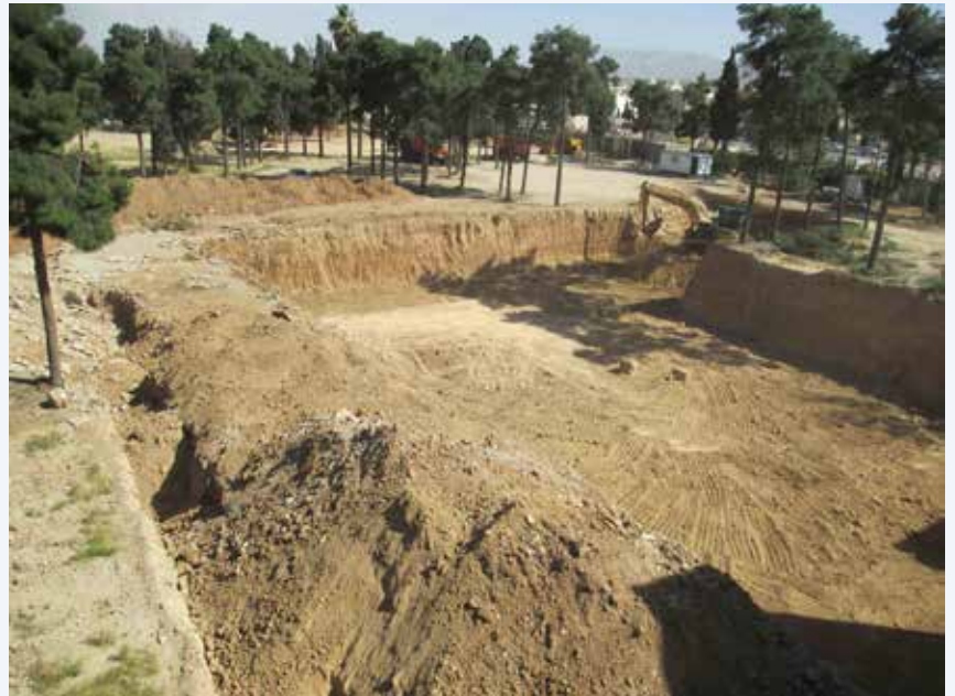
In early 2014, Revolutionary Guards dug this hole, allegedly for the foundation of a new cultural and sports center, in a historic Bahá'í cemetery in Shiraz.
